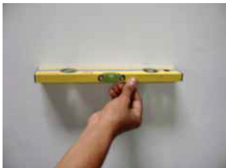
View B. Verify Horizontal Leveling
